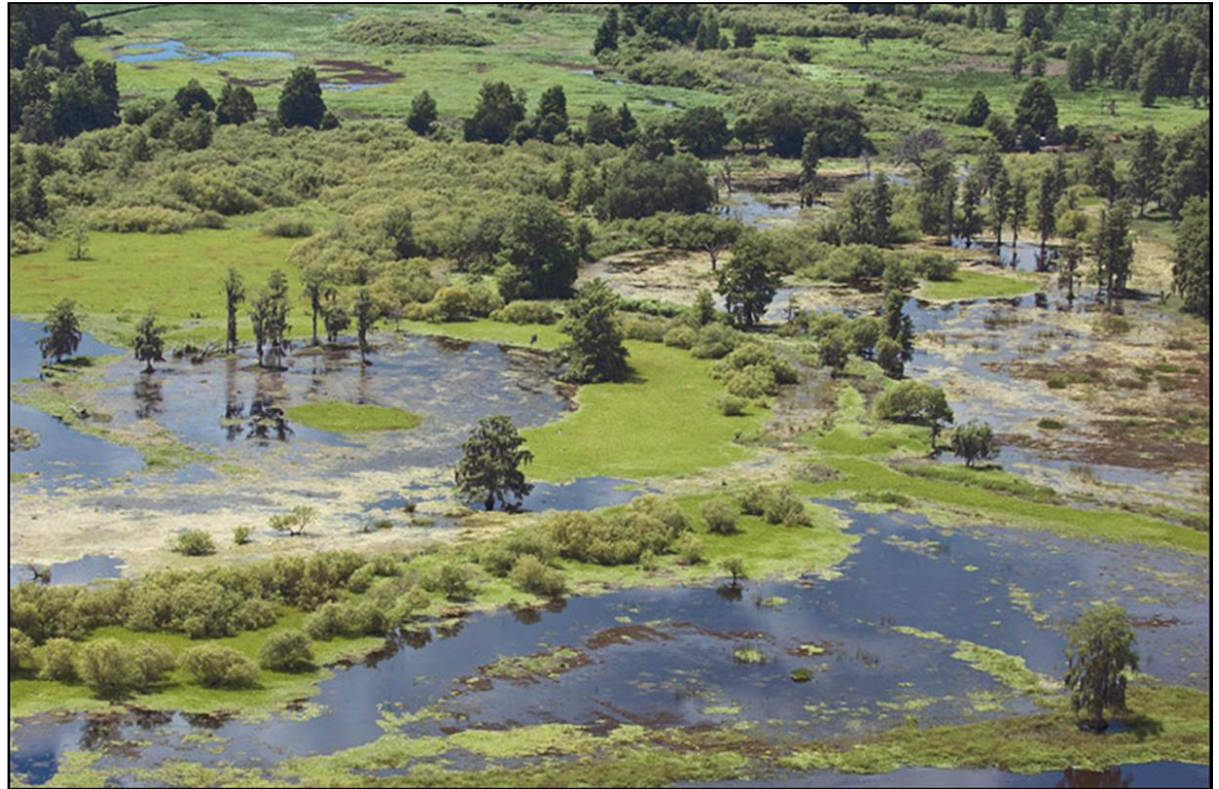
Dispersed Water Storage Site in the SFWMD
